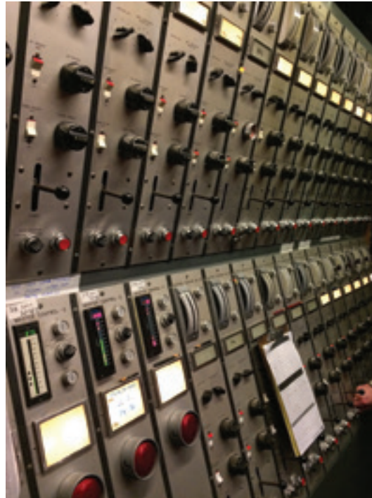
Metropolitan Opera, NY, flying control desk Courtesy of Jeff Mace, Metropolitan Opera
