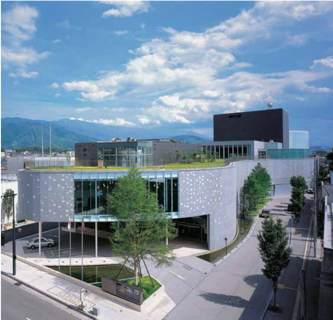
Exterior Courtesy of Matsumoto/ Mpac
